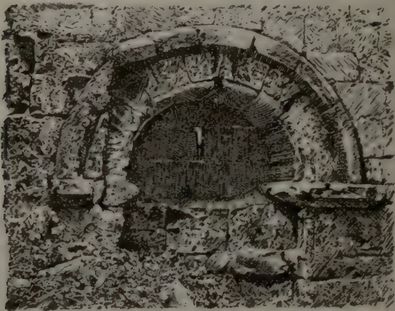
FIG. 10. DRAIN IN NORTH TRANSEPT.
